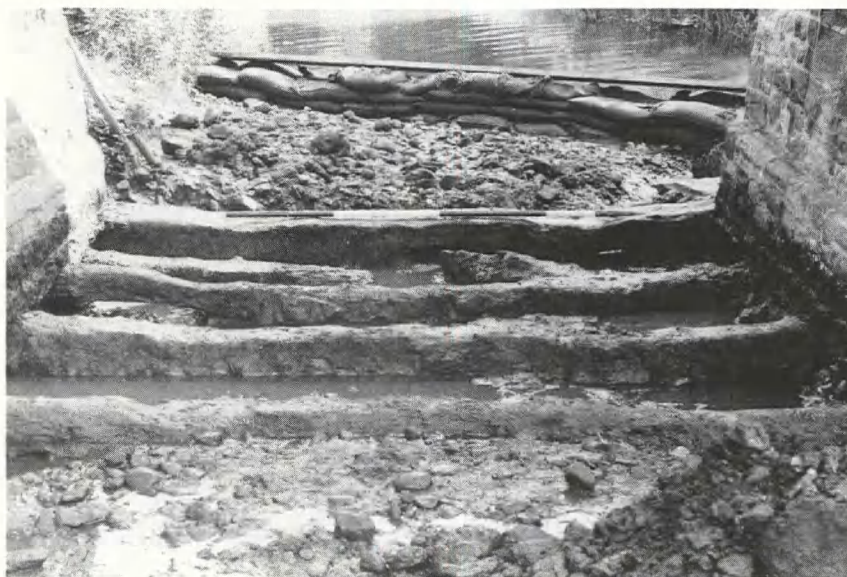
Plate 4 Elm raft, west arch from south, 1986
